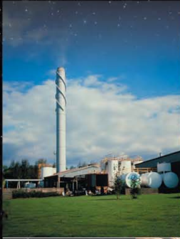
Ecology (Recycling Facilities)
